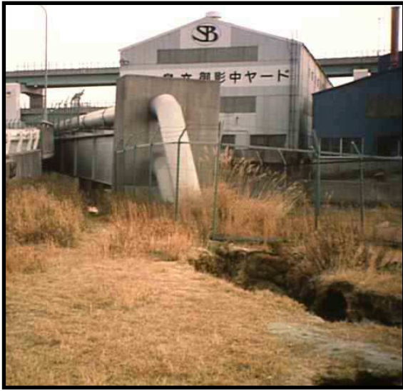
Photos 1A and 1B showing ground cracking due to liquefaction/lateral spreading in the vicinity of Osaka Bay, and a pulled joint in a ductile iron pipeline (Kobe 1995).
