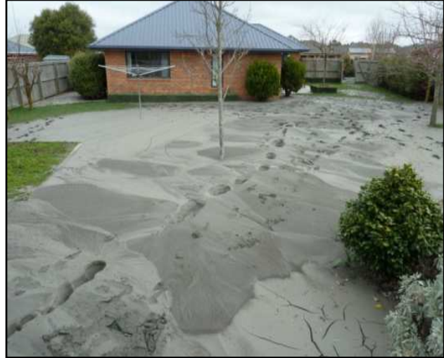
Photo 2. Ejected liquefied sand along the Avon River in Christchurch (New Zealand, 2011) (Photo by Tonkin & Taylor)
